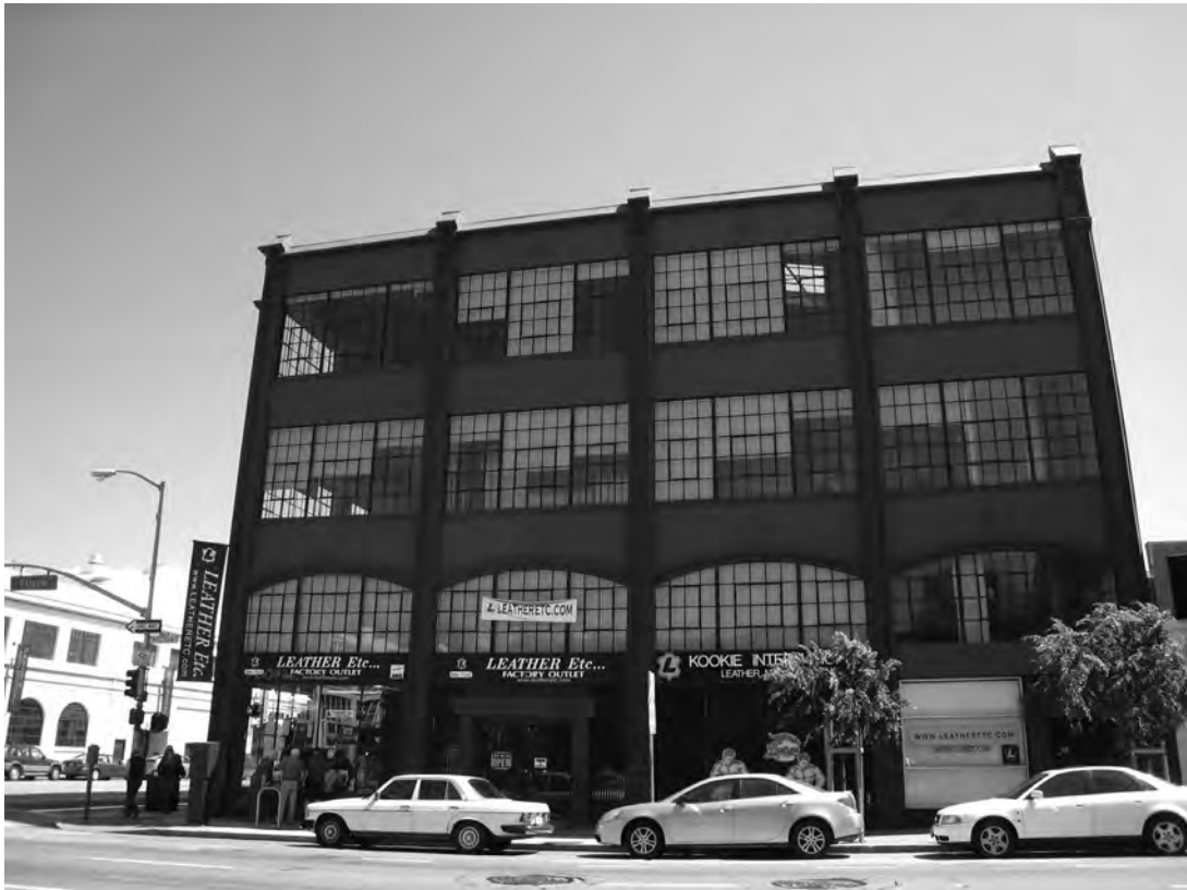
Commercial building at Eighth and Folsom Streets
